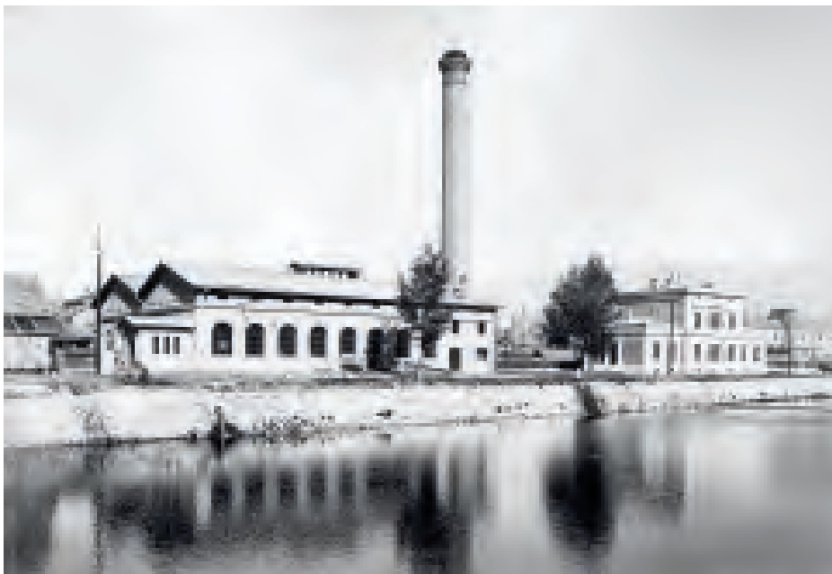
Kraftwerk an der Hiseta-Straße. Siemens Corporate Archives, München / The new power station on Hiseta Street. Siemens Corporate Archives, Munich
